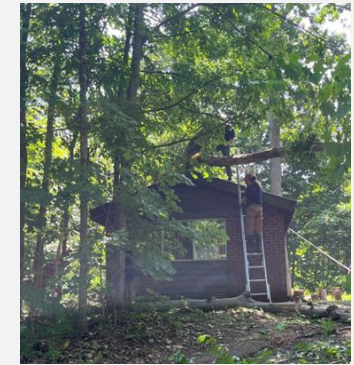
Canada: Renovation at summer camp for underprivileged children
