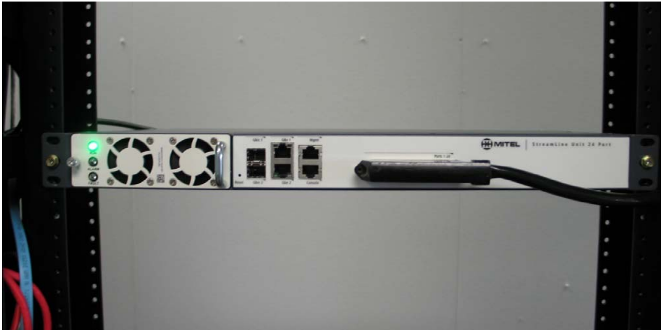
Figure shows the Mitel StreamLine installed in a standard 48 cm (19") rack.
