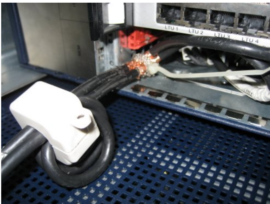
Figure 45: Closed ferrite core with DC cables
