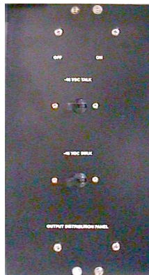
Figure 202: Output distribution panel, front view
