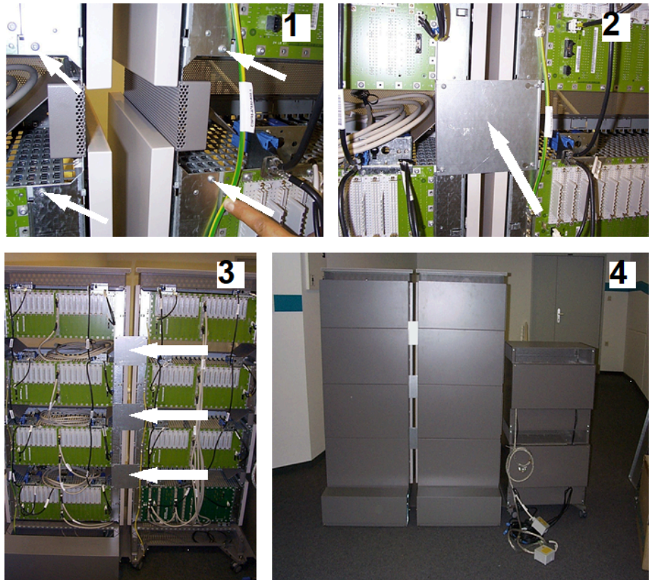
Figure 81: Installing the ground straps between the cabinets
