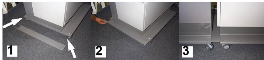
Figure 80: Installing the ground strap at the base of the cabinets
