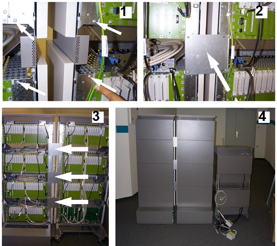
Figura 114: Colocar as juntas de terra entre as caixas
