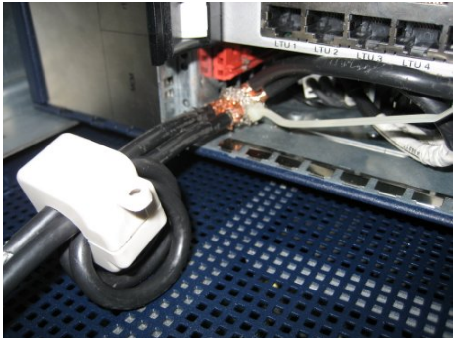
Figure 47: Closed ferrite core with DC cables
