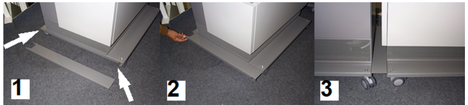
Figure 82: Installing the ground strap at the base of the cabinets
