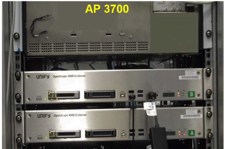
Figure 63: Example of 19" installation with EcoServer (duplex) and AP3700
