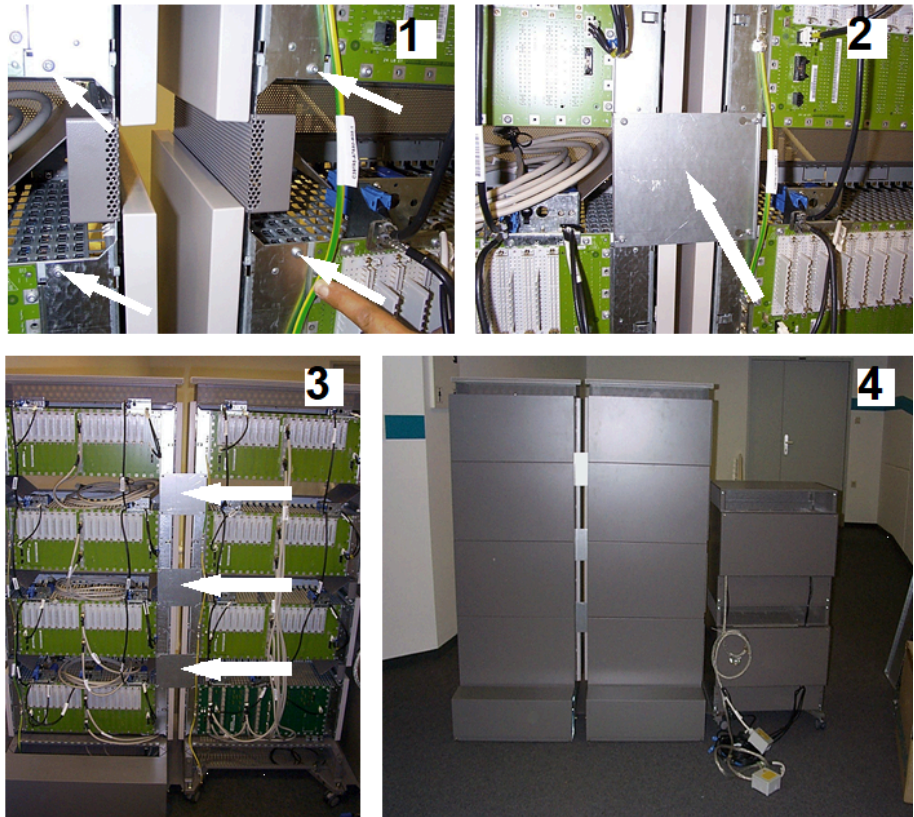
Figure 83: Installing the ground straps between the cabinets
