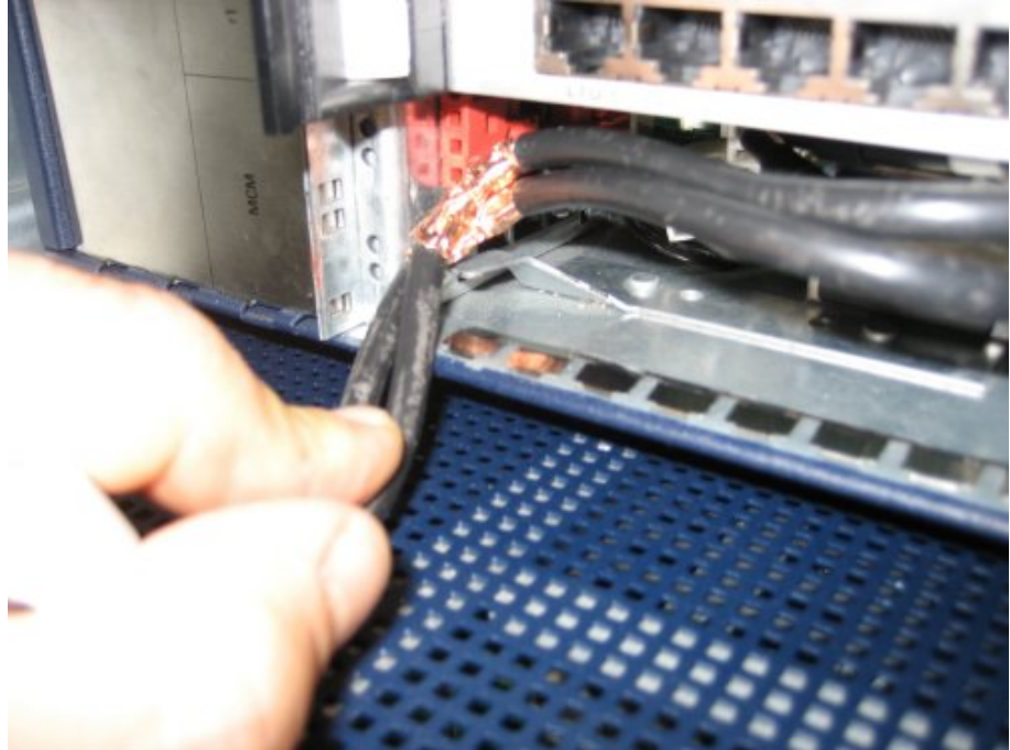
Figure 42: Stripped DC cable
