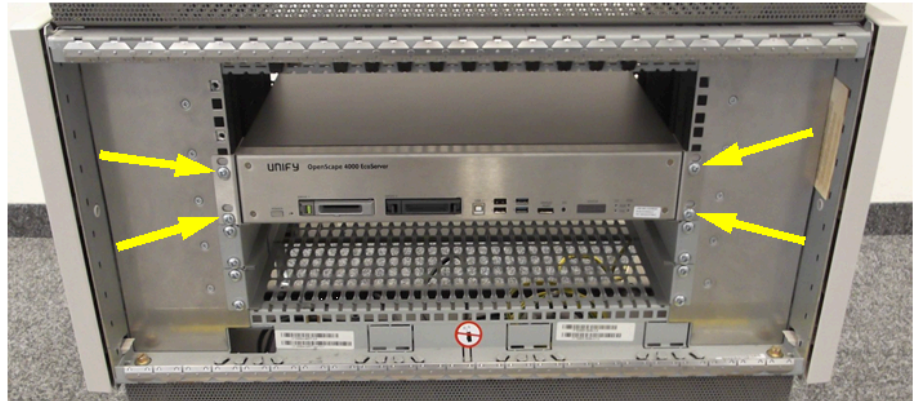
Figure 26: Installing the EcoServer
