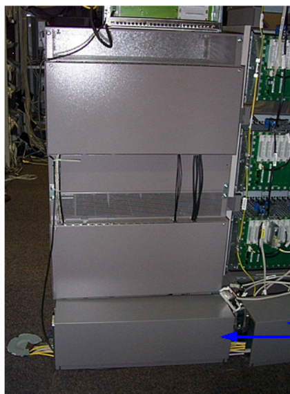
Figura 241: Colocar as tampas do canal de cabos
